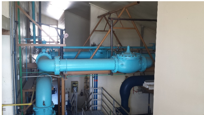
Filter Backwash Piping
